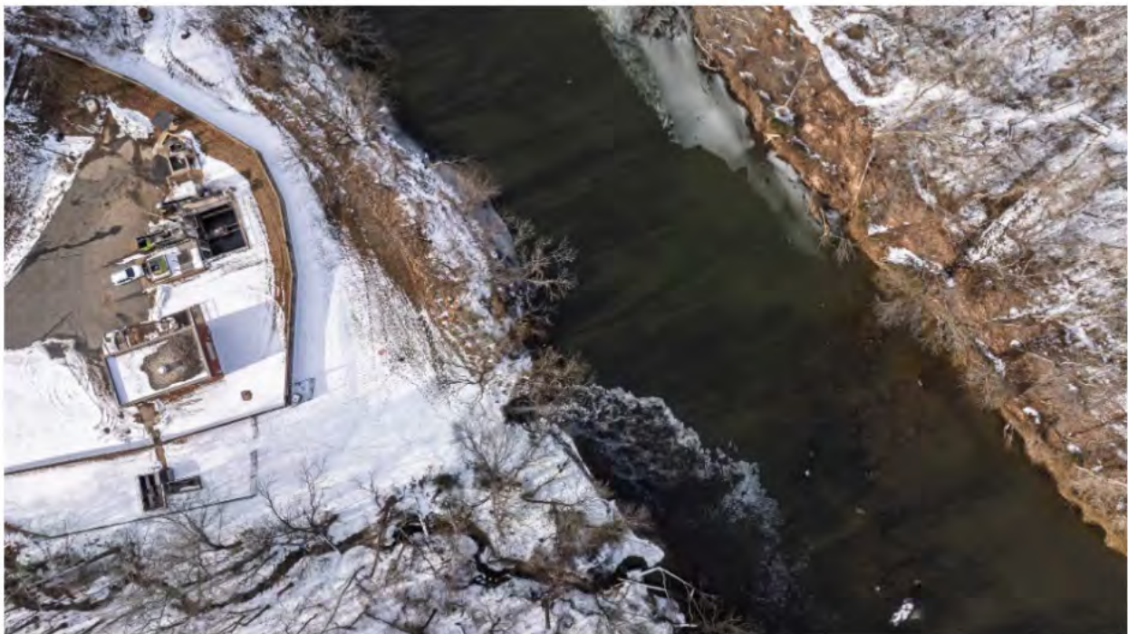
The East Burlington Wastewater Treatment Plant's outfall (visible just above the creek in the photo) discharging treated effluent to the Haw River in winter.
