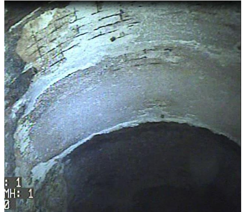
Concrete Sewer Main less than 40 years old
