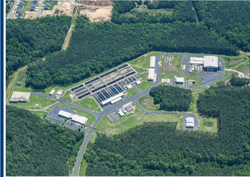
Western Wake Regional Water Reclamation Facility (18 MGD Capacity)
