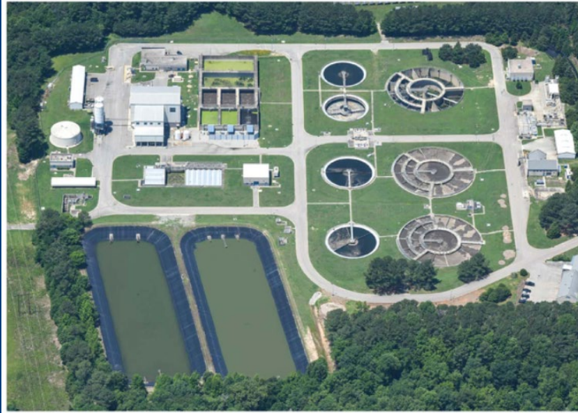
South Cary Water Reclamation Facility (12.8 MGD Capacity)
