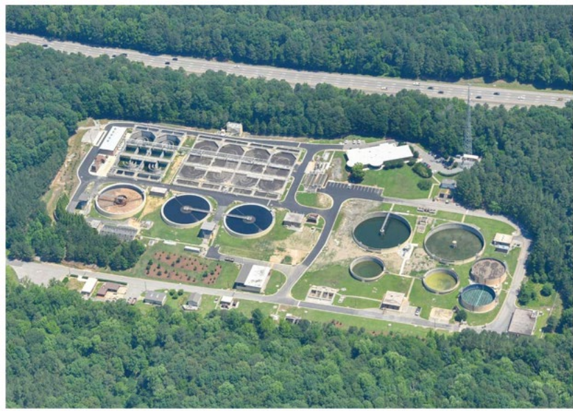
North Cary Water Reclamation Facility (12 MGD Capacity)
